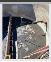
Chuck explained that the picture on the left is SBR#3 before it was cleaned out and the one on the right is after it was cleaned out and before the decanter was put back in.
